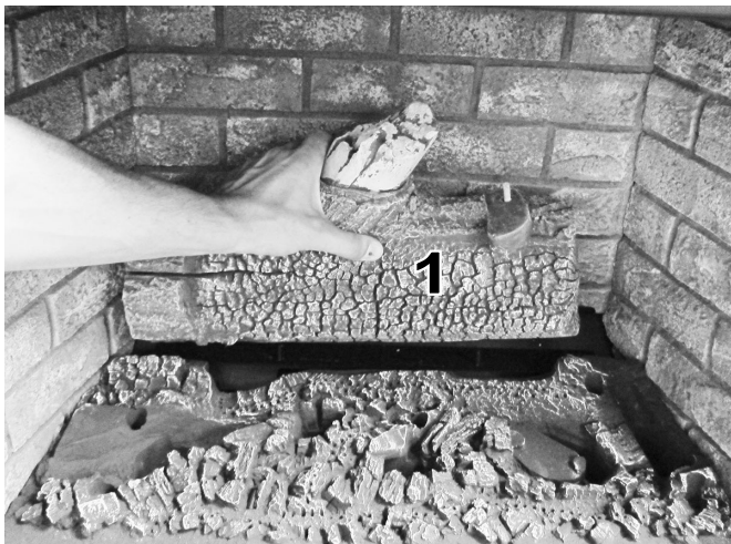
Figure 35. #1 Log. Engage the two pegs located on rear burner skirt with the holes in the underside of the log.
